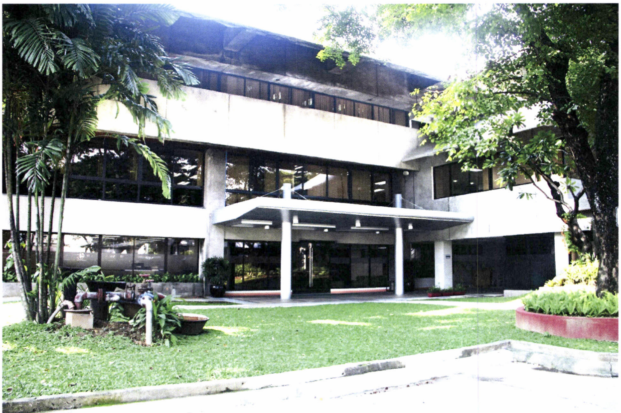
TransCo Main Building, Power Center, Quezon City
